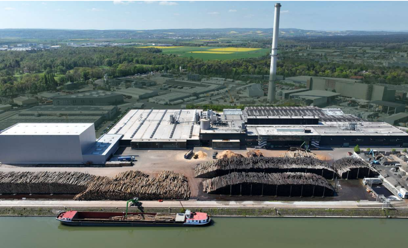
The production site in Aschaffenburg is Europe's largest solid wood cutting plant.
